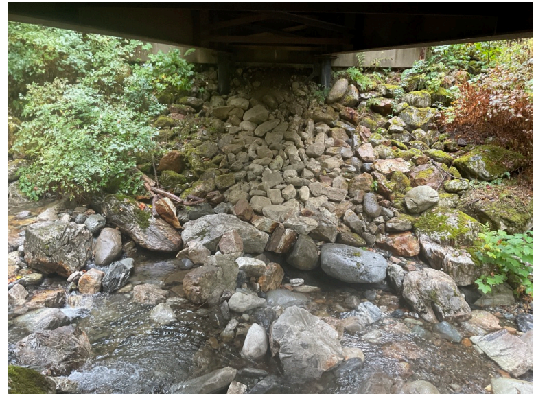
Left Bank Abutment when facing downstream
