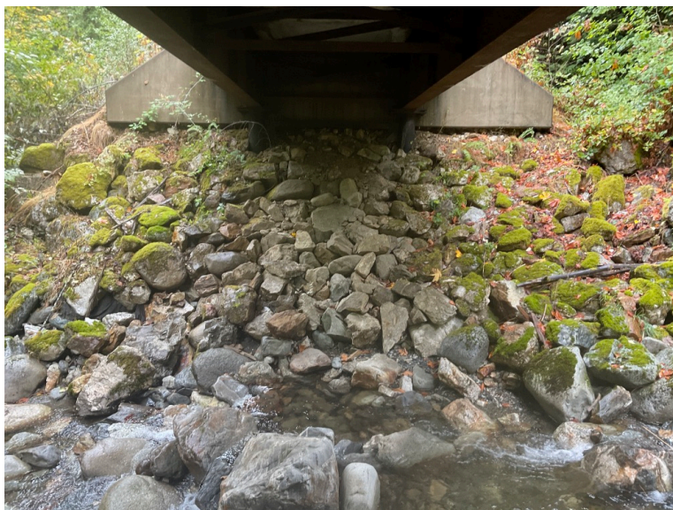
Right Bank Abutment when facing downstream
